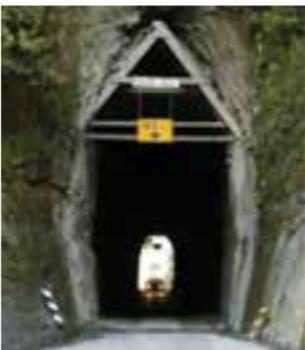
The single-lane 180m long **Moki Tunnel** was built in 1936 and is known locally as the 'Hobbit's Hole'. Home to fossilized giant crabs, the tunnel's floor was lowered in 1989, increasing the tunnel's height to 7m to allow access for triple-decked stock trucks. It has a timber gabled roof and hand carved walls.
